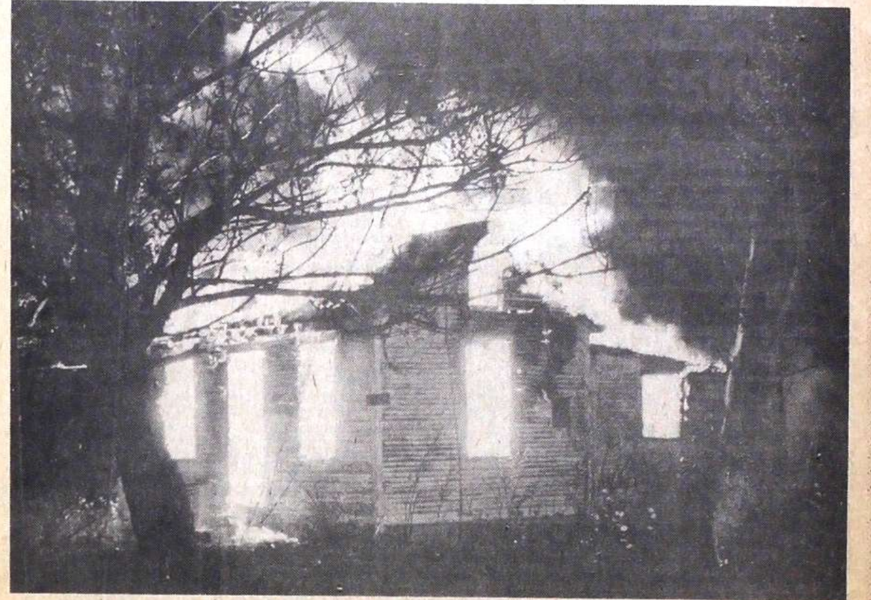
VACANT HOME BURNS —A fire of undetermined origin swept through a vacant home in Romulus Monday night, leveling the structure. The fire in the home at the corner of Heyer and Van Born Roads began about 10:30 p.m. Romulus Fire Chief Joe Crova said he had no idea how the fire started.
